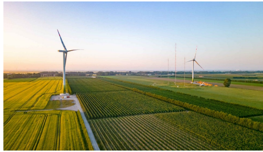
Figure 1: Wind turbine at the DLR research wind farm WiValdi.
