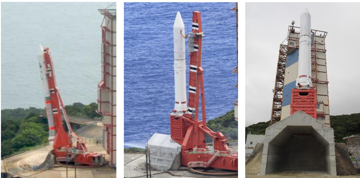
Fig. 1. USC Launch Pad. Before Refurbishment for M-V Vehicle (left) and Present Structure for Epsilon (middle and right).
